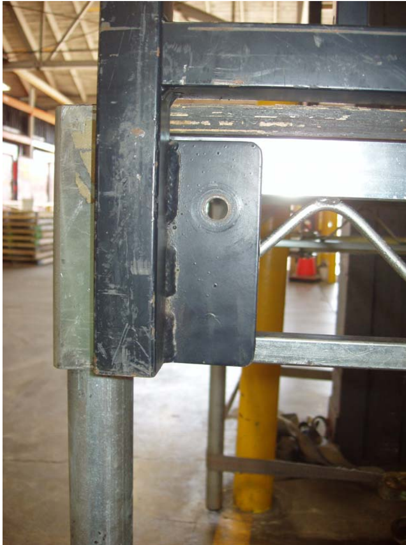
Figure 3-9 Guardrail bottom joint after tests #1-3
