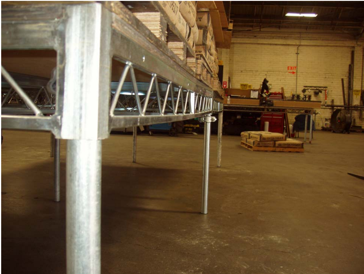
Figure 3-3 Load Step 2, 1 st Stage loaded to 271.0 lbs/ft 2 , Sag of long side beams
