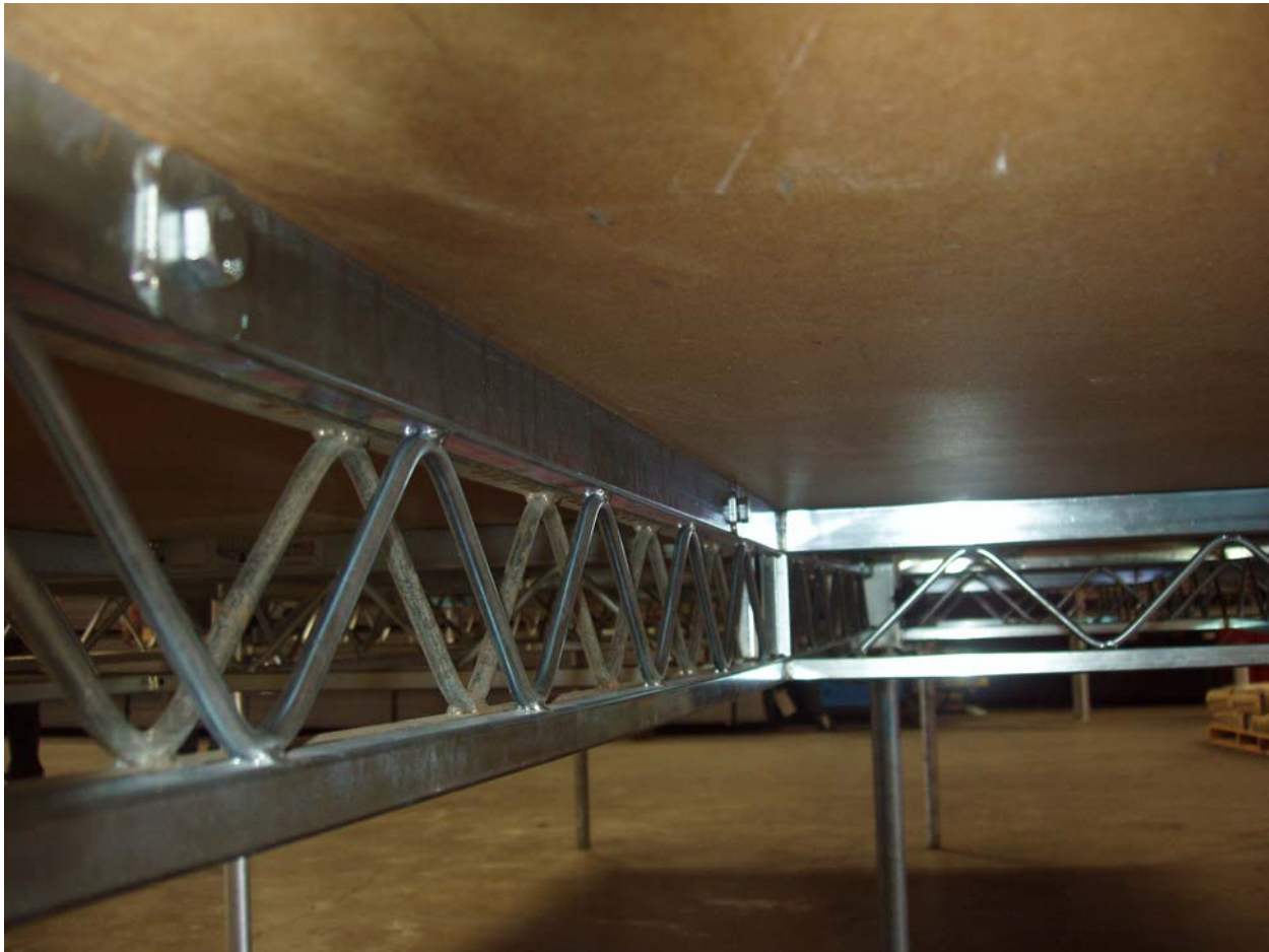
Figure 3-5 Load Step 2, 1 st Stage loaded to 271.0 lbs/ft 2 , Inboard long beams
