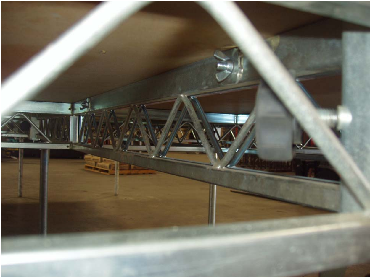
Figure 3-4 Load Step 2, 1 st Stage loaded to 271.0 lbs/ft 2 , Inboard long beams
