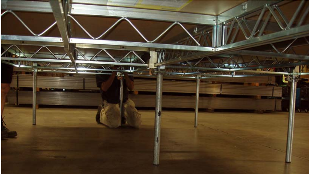
Figure 2-2 Test Stage, View from below of Critical Central Leg
